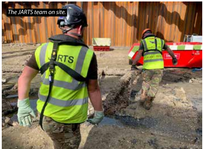
The teams worked inside the Cofferdam structure.
